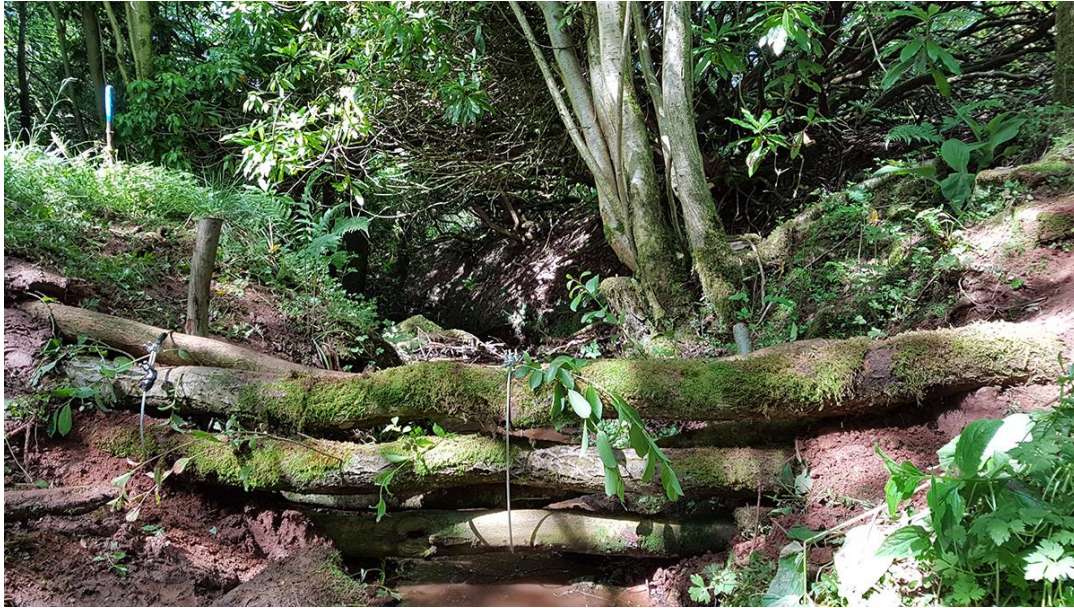
Figure 39: Example of a Small-Scale Leaky Weir
